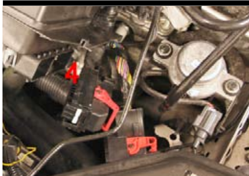
4. Remove the connectors (4) from the ECU. Loosen both of the red clips and pull the connectors. Remove the electrical harness from the air filter box. Cut the tie wraps (4pcs) from the harness.
